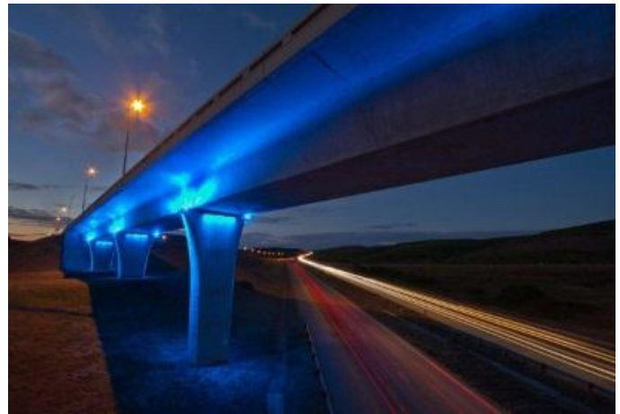
N2 Bridge – Pictorial (Open)
